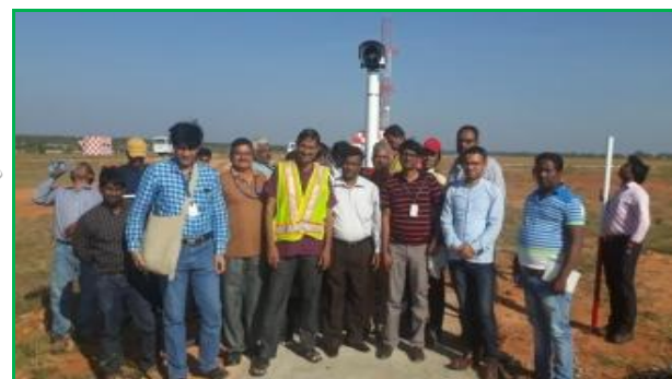
Installation of "Drishti RVR"
