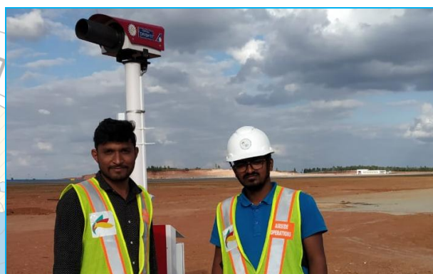
Installation of Drishti-AWOS
