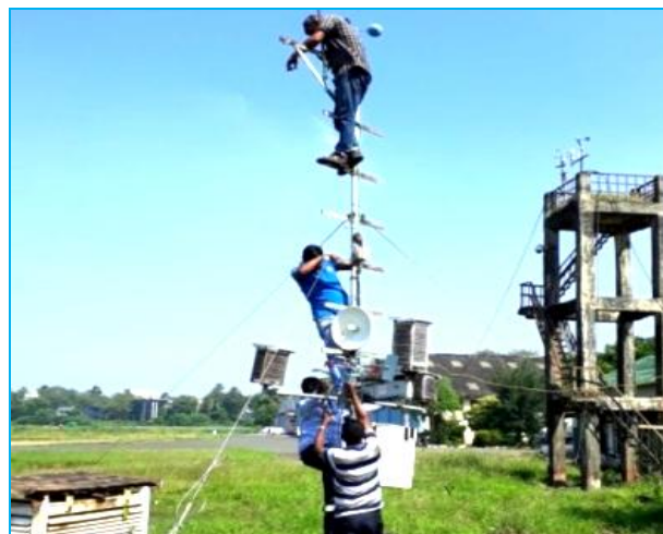
Integrated PC based Software System to DCWIS system
