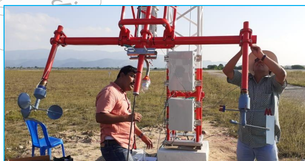
Installation of DCWIS system
