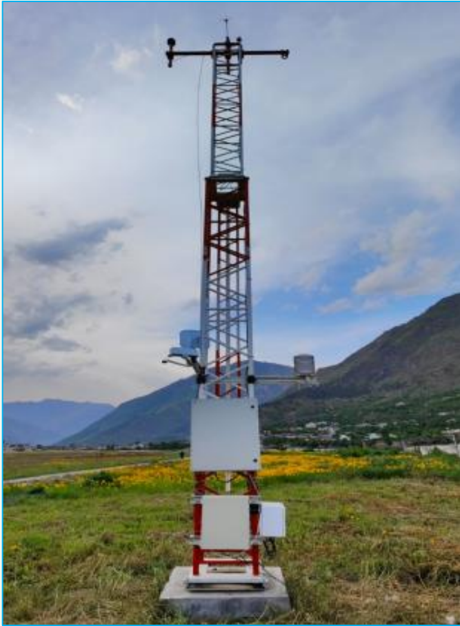
DCWIS and PWD systems
