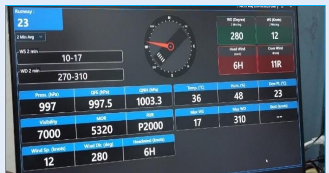
DCWIS & PWD at Keshod Airport
