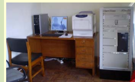
DMDD receiving system at Kathmandu
