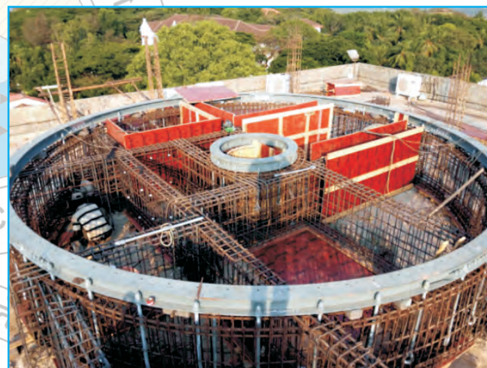
Doppler Weather Radar building under construction at Goa
