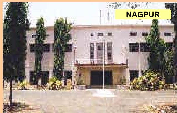
Regional Meteorological Centre, Sonegaon Aerodrome, NAGPUR - 440 005
