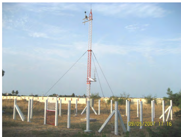
AWS installed in the premises of CDR, Karaikal, Tamil Nadu
