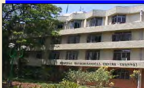
Regional Meteorological Centre, Chennai
