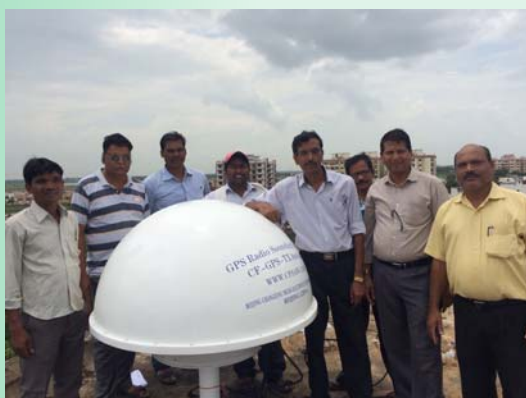
Antenna Installation of Radiosounding system
