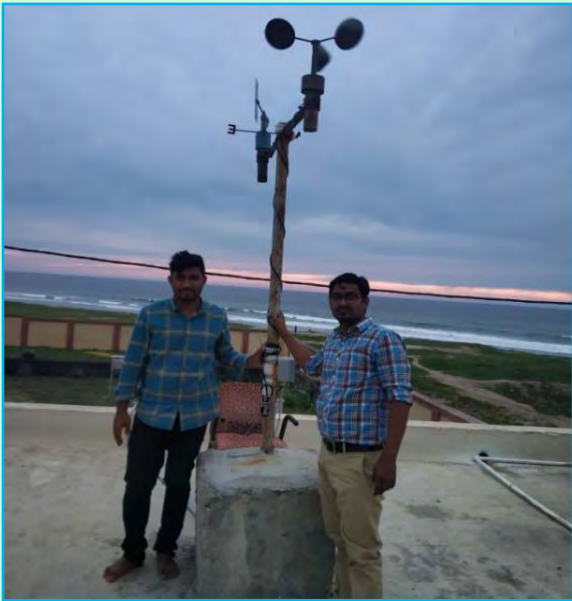
Fig. 15. HWSR installed at Veraval
