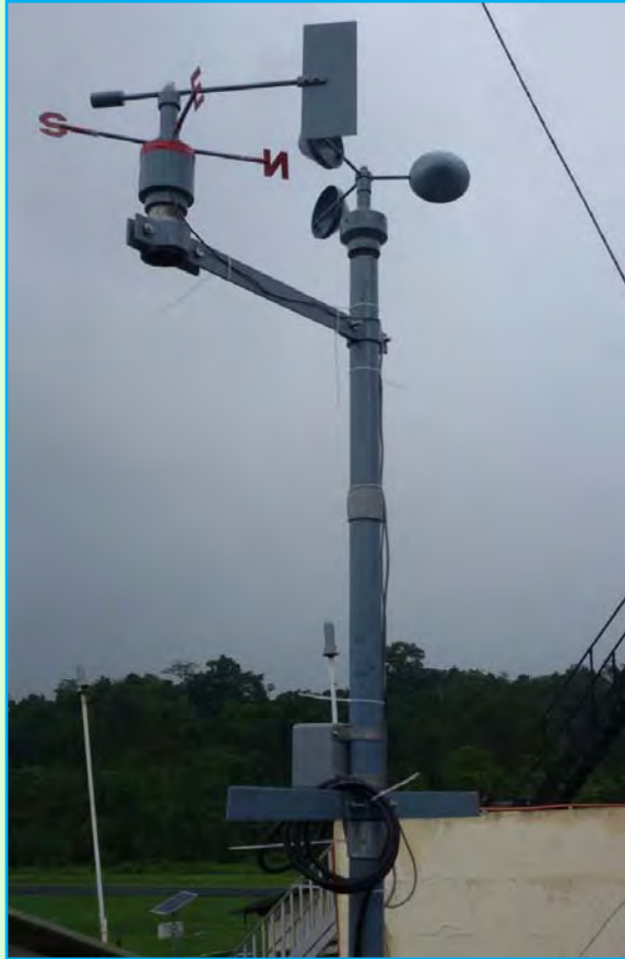
Fig. 13. DIWE System installed at Port Blair
