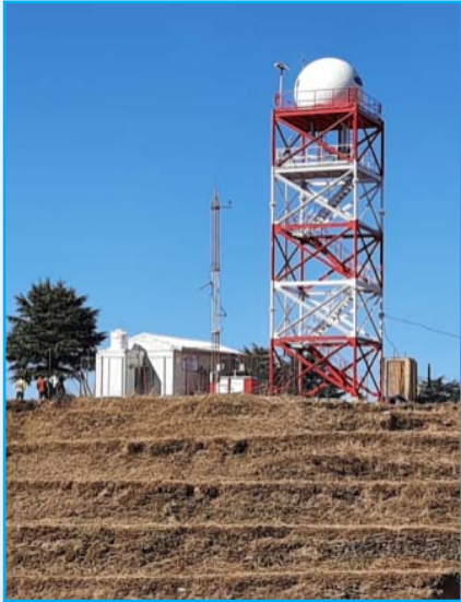
DWR at Kufri in Himachal Pradesh
