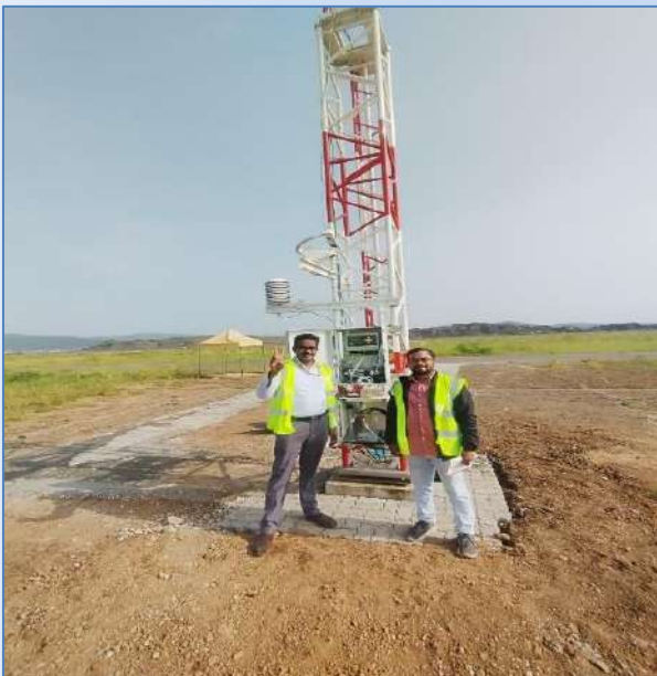
Installation of Two DCWIS and five RVR systems at Navi Mumbai airport
